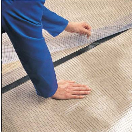
Joining vapour barrier membranes
