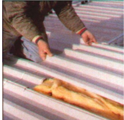
Sealing lap joints in industrial roofing
